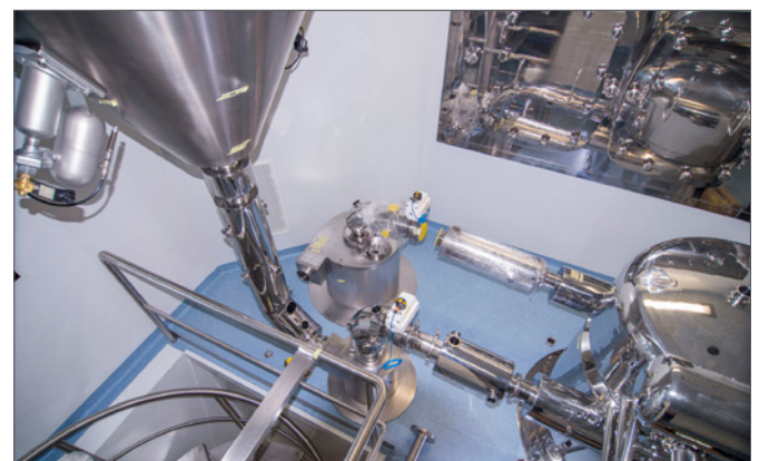
Fig. 2 - Installation of a similar hurricane cyclone at Hovione
